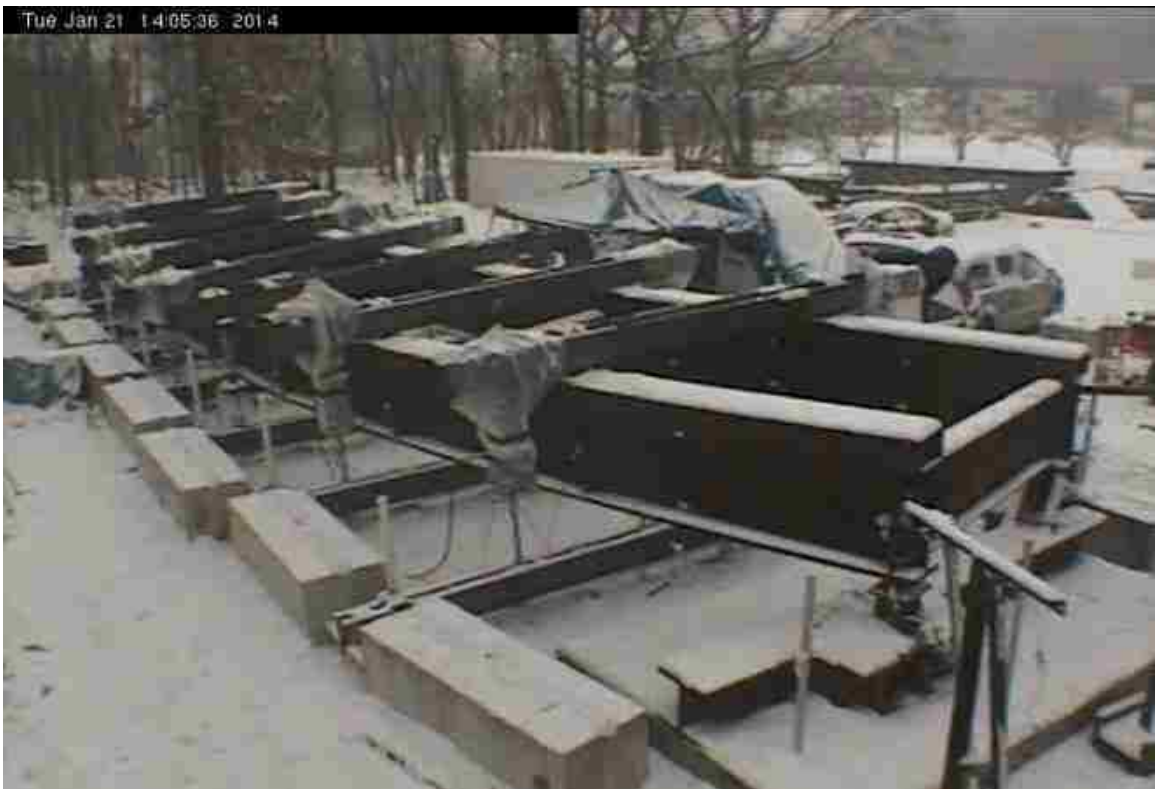
Figure 7.6 Test specimen condition at load step 17 of the inelastic test
