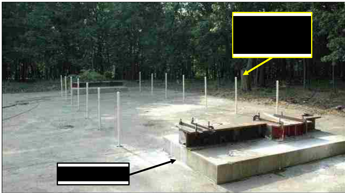
Figure 2.11 Installed ground anchor rods covered by plastic pipes (Sause et al., 2009)
