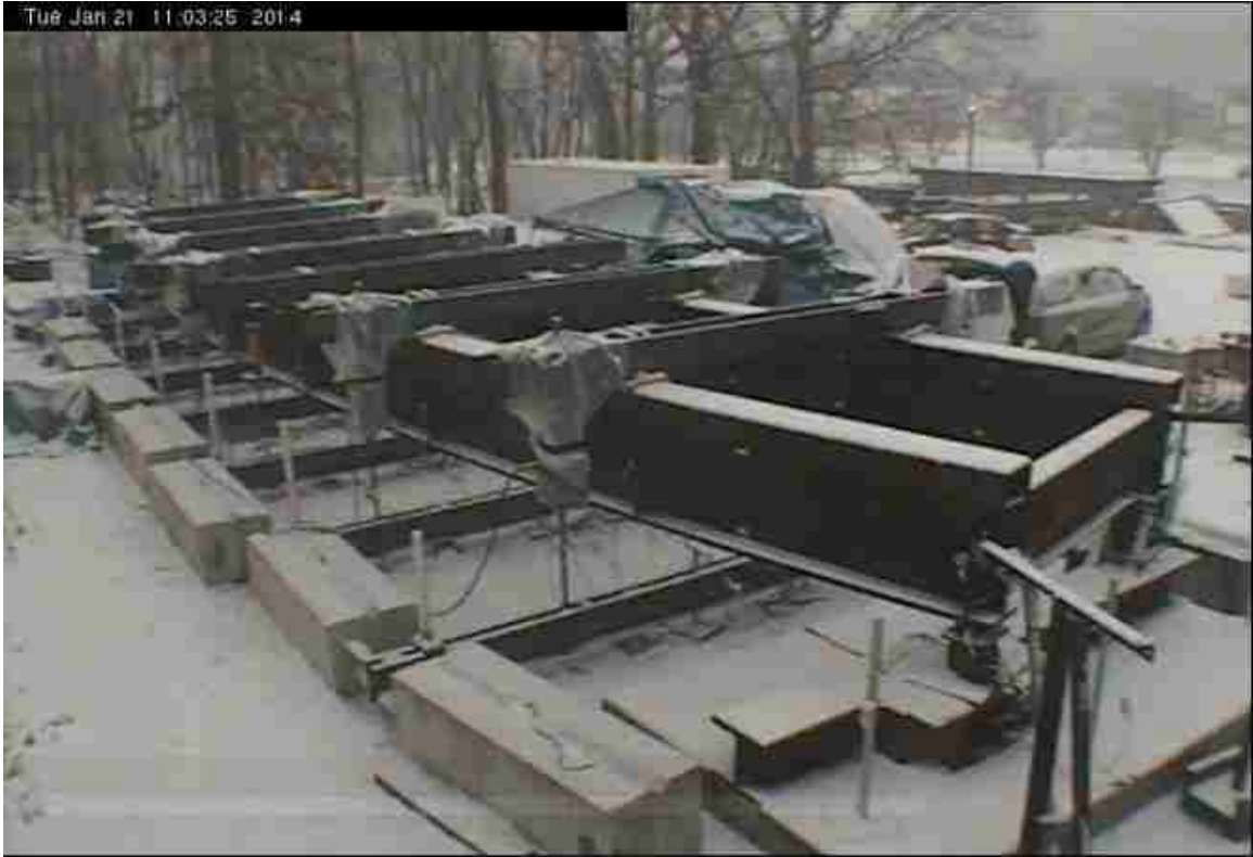
Figure 7.5 Test specimen condition at start of the inelastic test
