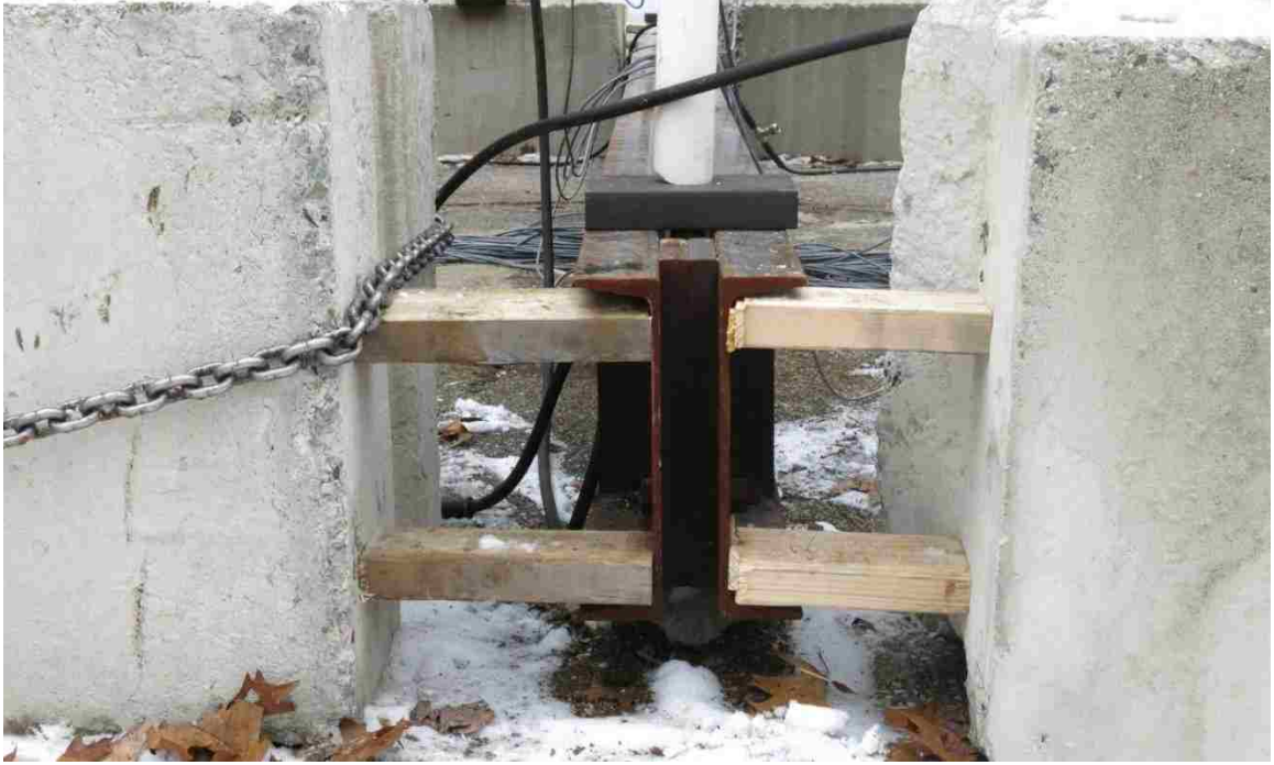
Figure 3.22 Photograph of concrete blocks and wooden wedges bracing load transfer channels
